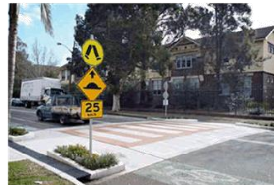
Raised crossing slows traffic and improves pedestrian safety and visibility
