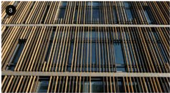
Building C: Enlarged existing commercial The existing commercial floorplate will be enlarged to approximately 1,600sqm (GLA) and clad with external blades to soften the materiality of the existing building and respond to the human scale at its low height.
